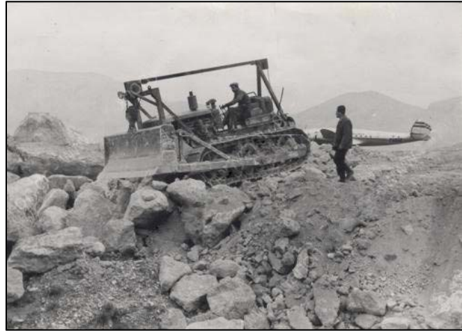
Figure 4.3 A snapshot of the airport’s expansion in 1957.
